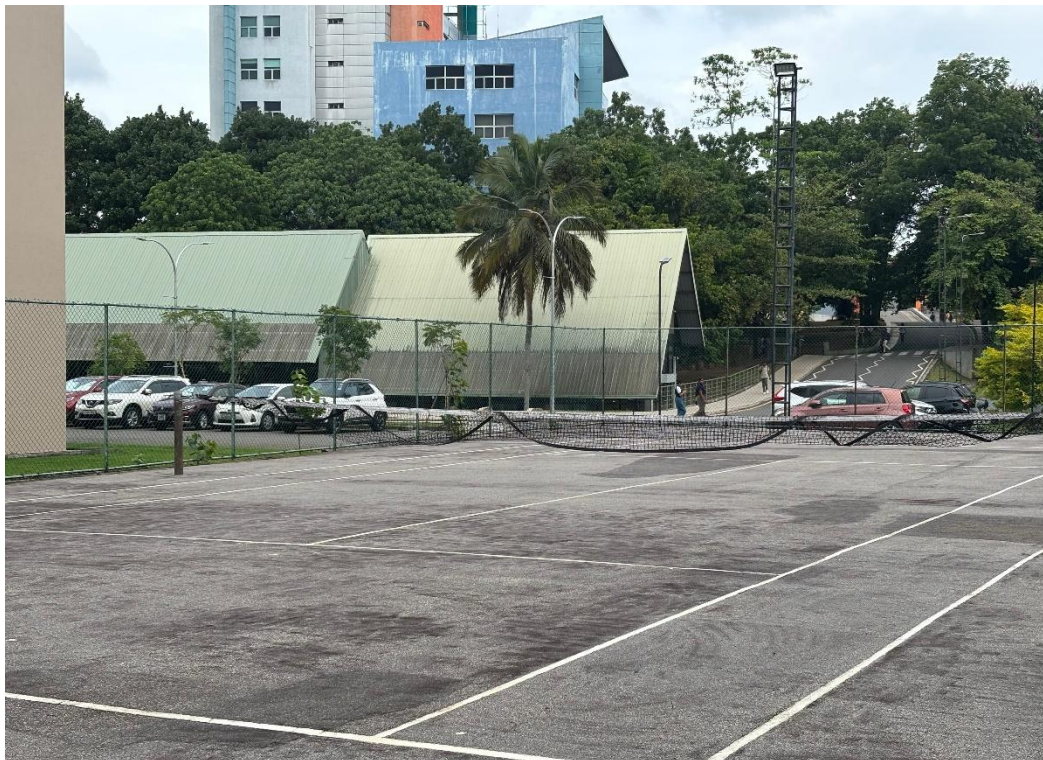
Figure 4: View of Block AC
