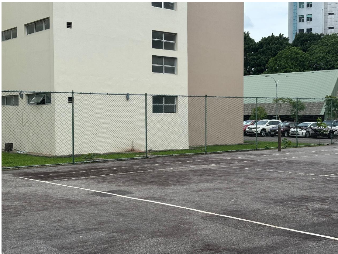
Figure 10: View of Block A
