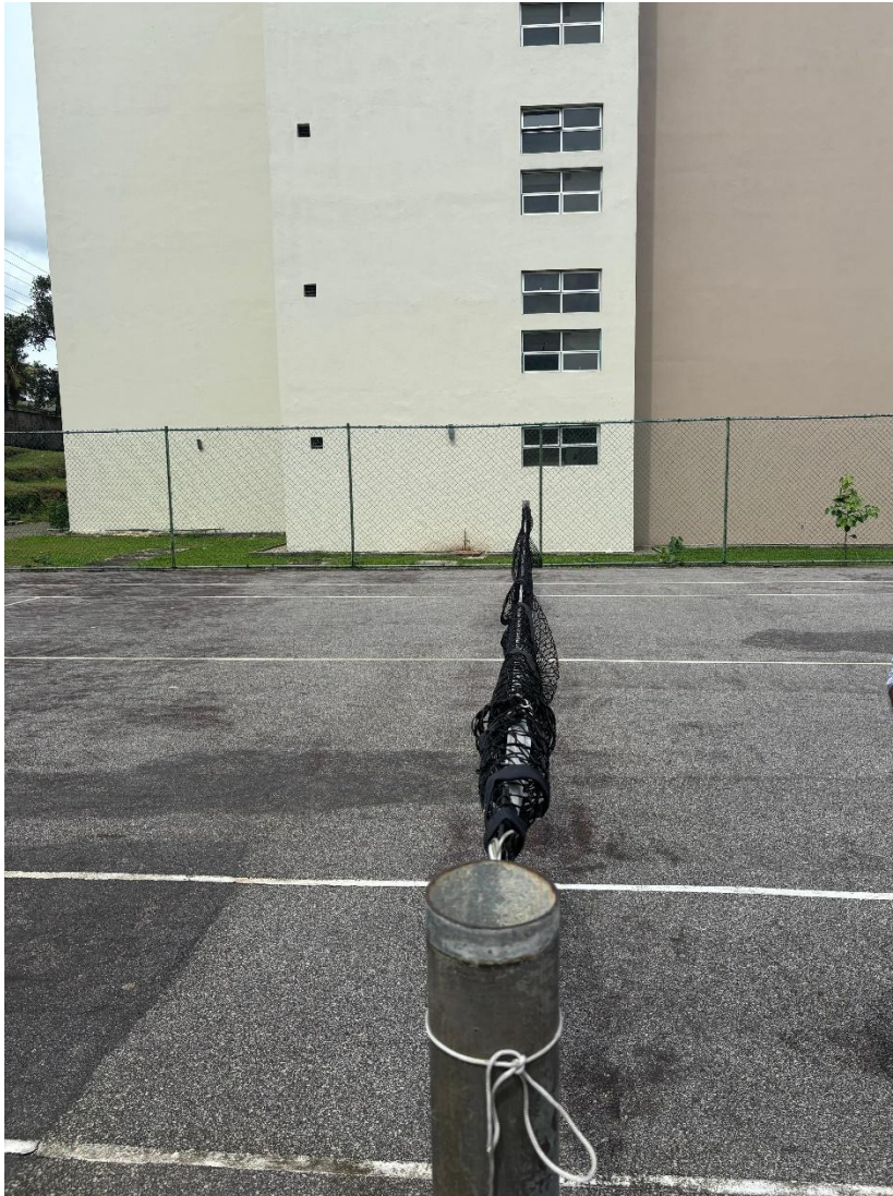
Figure 11: View of Block A
