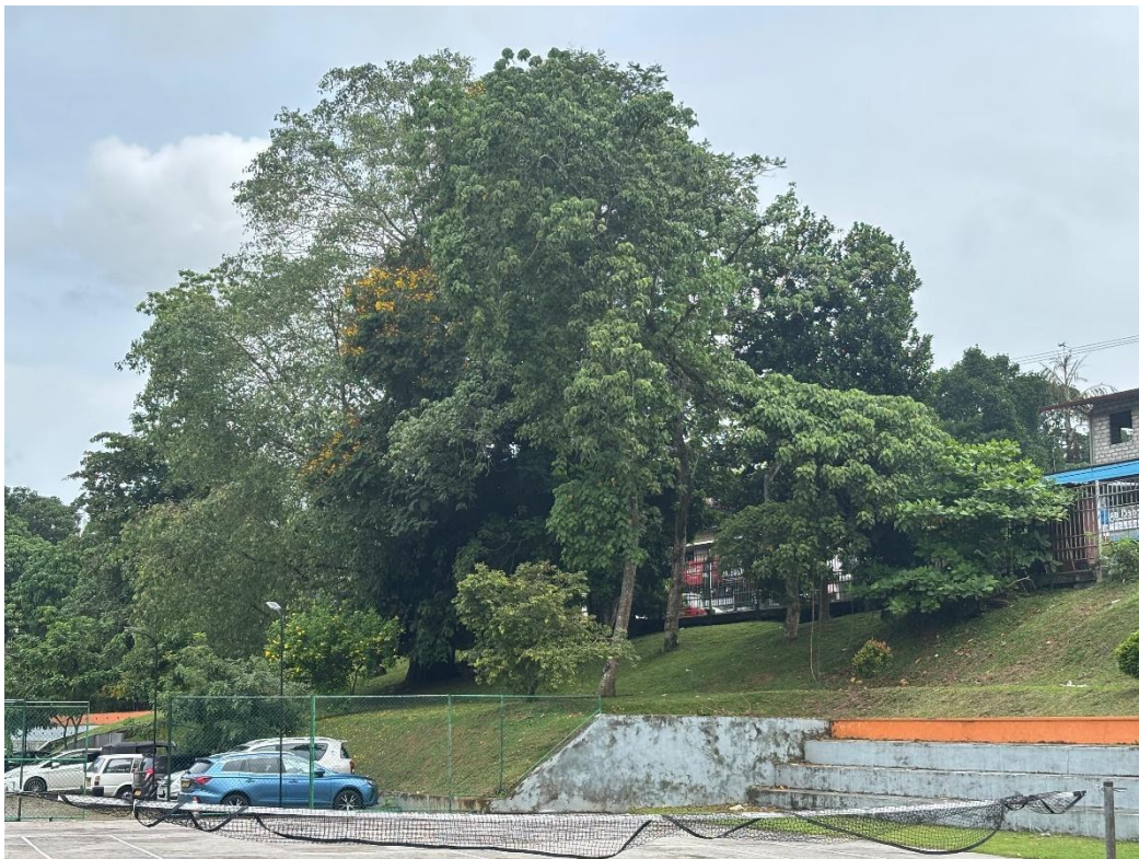
Figure 7: View of Block BC
